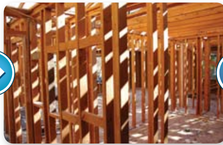
Walls carefully stripped to the studs
