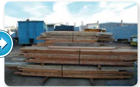
Studs from the old home stacked and ready for reuse
