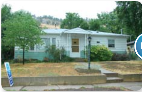
Existing 1,000 sf home prior to deconstruction
