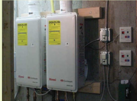
Units can be installed in tandem to increase hot water supply.
