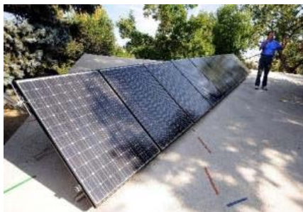
The solar installation at the home of Thomas David Kehoe was done poorly according to Kehoe. He is showing that the panels are shaded by trees much of the day. ( CLIFF GRASSMICK )
