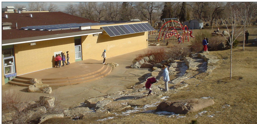
Below: 10 kilowatt photovoltaic system donated to Flatirons Elementary by ReNew Our Schools program and installed by Bella Energy.
